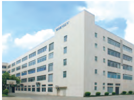
R&D Center in Guangzhou
